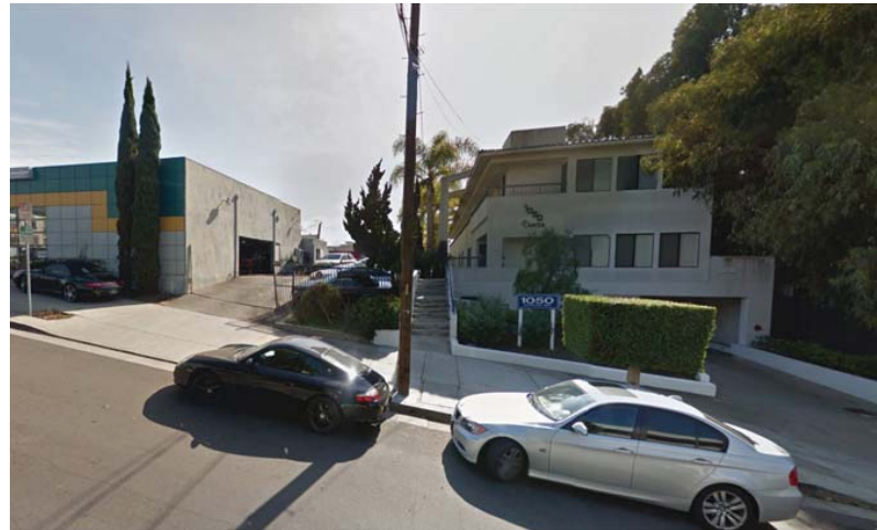
Photo 12: Looking south at 1050 Duncan Avenue
