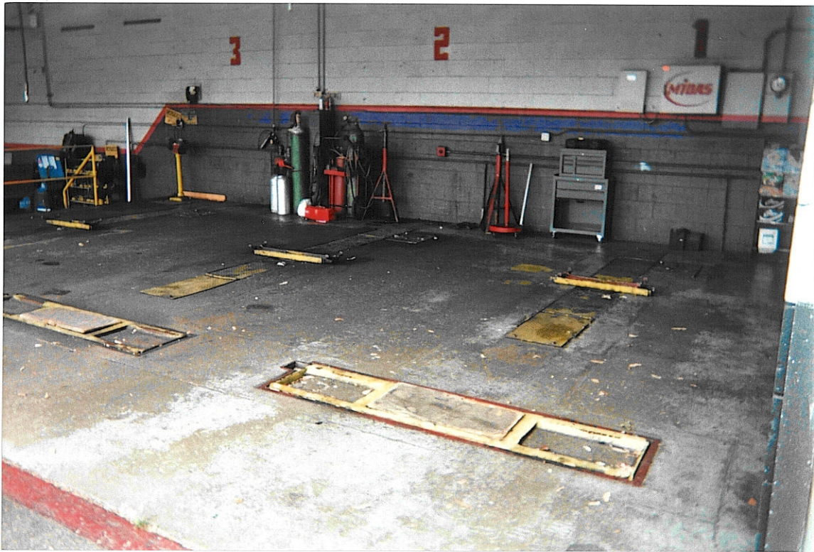
PHOTOGRAPH 3 – View looking west at service Bays 1, 2, and 3. The office area is to the right of the view. Each bay has an in-ground front-to-rear lift with a vault. The rear piston (in the foreground) is stationary. The front piston moves back and forth in an 8-foot deep concrete vault under the yellow steel plates. The front piston is under the yellow steel arm that crosses the vault. Metal steps down to Bays 4, 5 and 6 is seen at the left rear.
