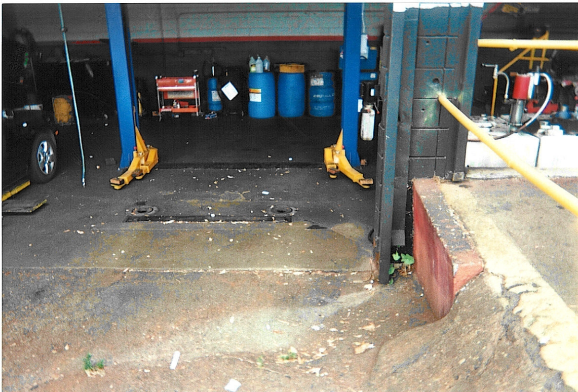
PHOTOGRAPH 4 – View looking west at Bay 5. An out-of-service dual-piston side-by-side in-ground lift is seen just inside the Bay. An above ground lift is behind the out-of-service lift. An operating side-by-side lift is present in Bay 6 to the left of the view. 55-gallon drums for new and used coolant and used oil filters are along the back wall. Bay 4 is to the right.
