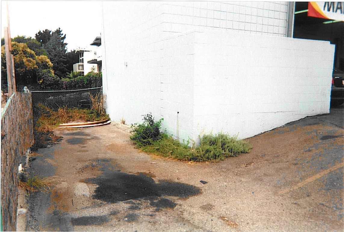
PHOTOGRAPH 5 – View looking west at the south side of the Site. The approximate 5-foot wide area is part of the vacated alley that is still present behind the houses in the distance. The vacant land beyond the fence appears to be part of a larger vacant lot south of the Site. A wall on the right is the trash enclosure at the corner of the building.
