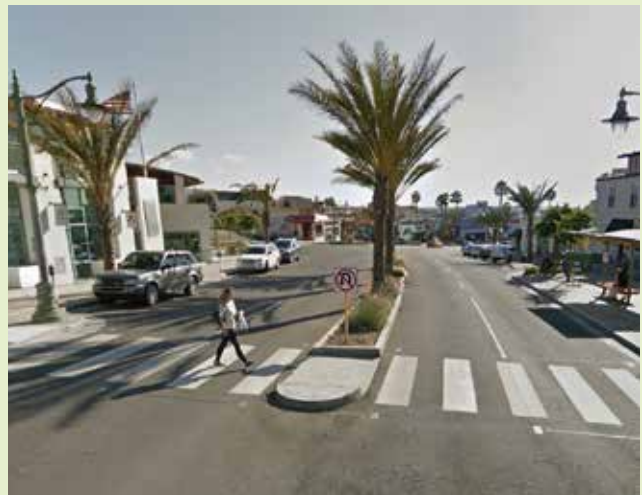
Upper Pier Avenue streetscape enhancements.
