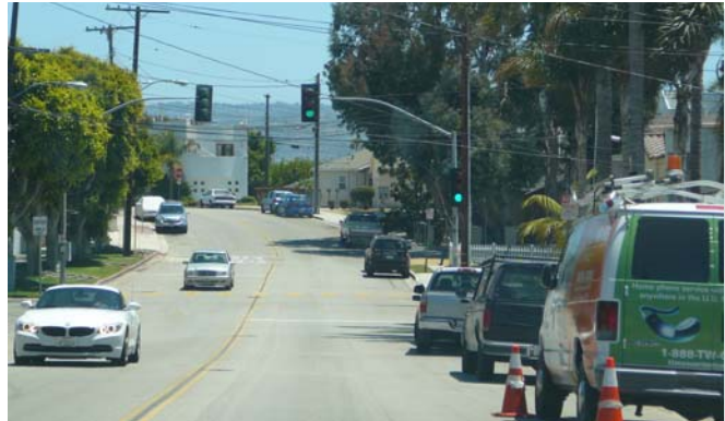
Bulbouts and high visibility crosswalks at intersection will visually narrow the road and reduce vehicle speeds.
