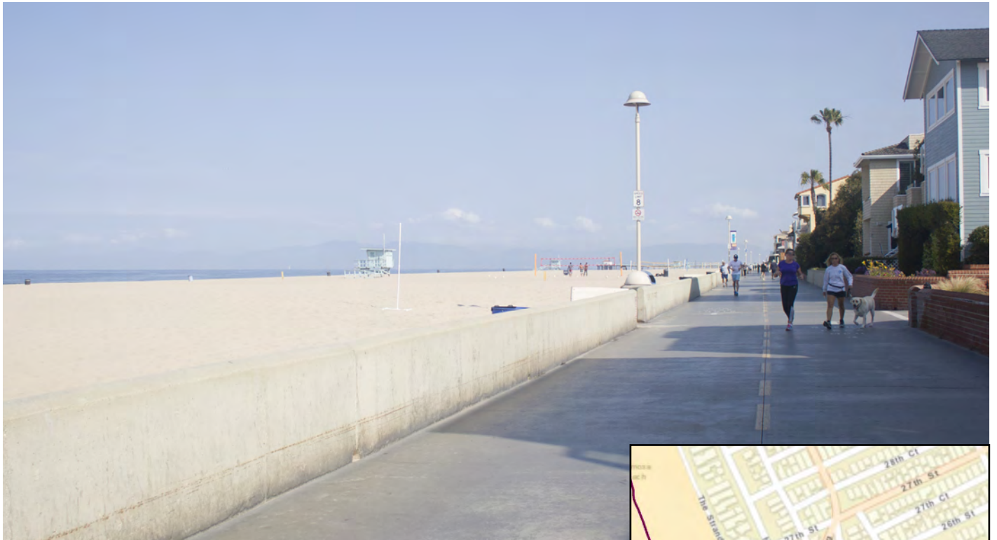
Existing Conditions- The Strand at 25 th Street looking northwest
