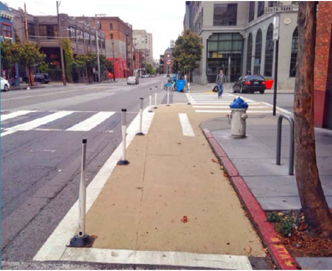
PAINTED CURB EXTENSION
