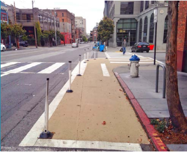
PAINTED CURB EXTENSION
