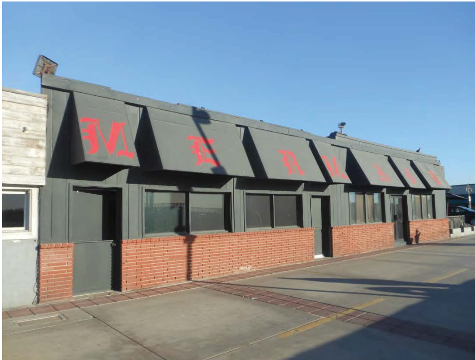
24. North side of 13 th Street, looking west
