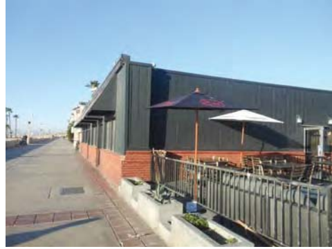
11 Pier Avenue, south & west elevation
