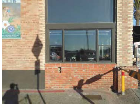
19 Pier Avenue, west elevation, window detail
