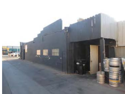
11 Pier Avenue, rear elevation (east)
