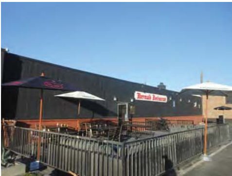
11 Pier Avenue, south elevation
