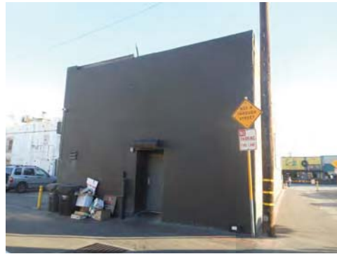
19 Pier Avenue, rear elevation
