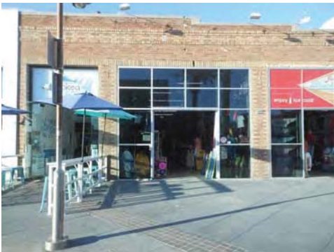
19 Pier Avenue, storefronts #4
