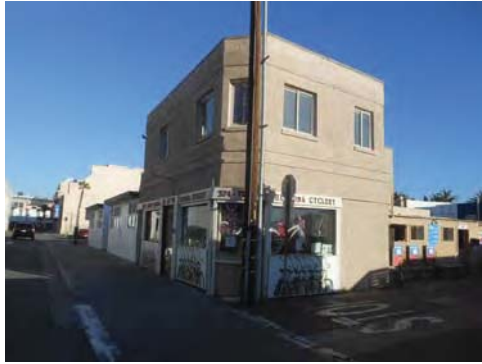
20 13 th Street, north & west elevations
