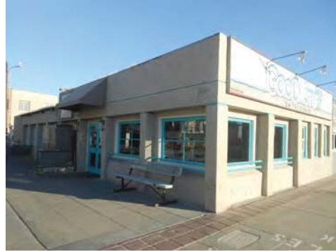
1272 The Strand, north & west elevations
