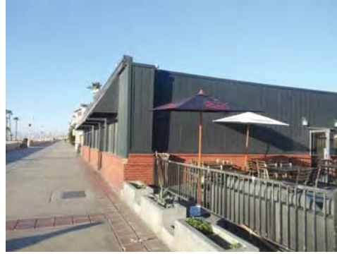
11 Pier Avenue, south & west elevation
