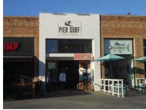
19 Pier Avenue, storefronts #2 & 3
