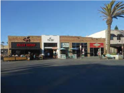
19 Pier Avenue, south elevation
