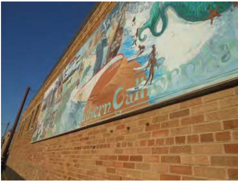
19 Pier Avenue, west elevation attached mural
