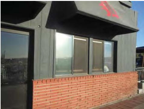
11 Pier Avenue, window & brick details
