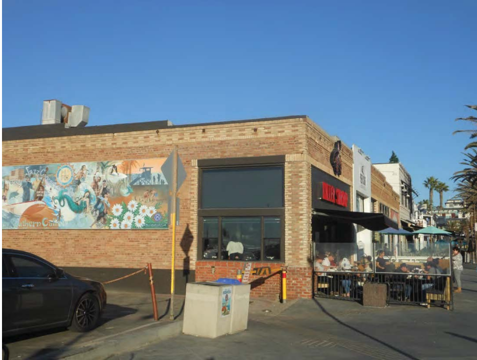
9. 19-31 Pier Avenue, west and south elevations
