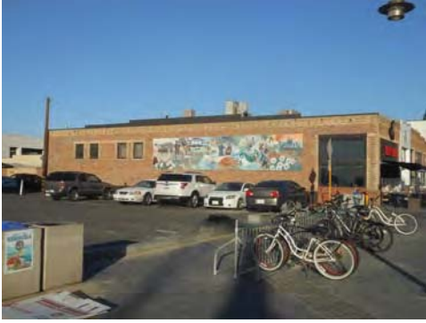
19 Pier Avenue, west elevation
