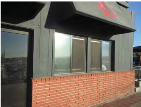
11 Pier Avenue, window & brick details
