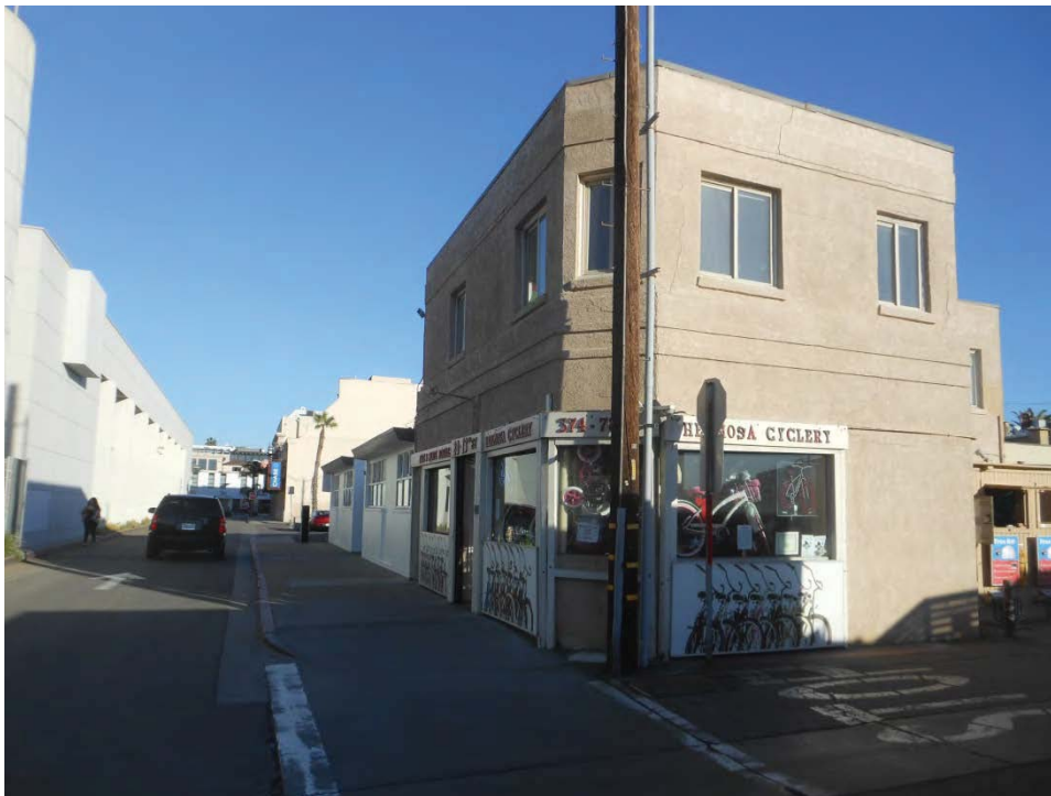
2. 20 13 th Street, north and west elevations
