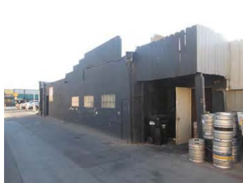
11 Pier Avenue, rear elevation (east)
