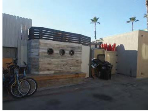
1250 The Strand, rear, east elevation
