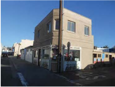
20 13 th Street, north & west elevations
