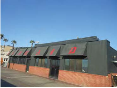
11 Pier Avenue, west elevation
