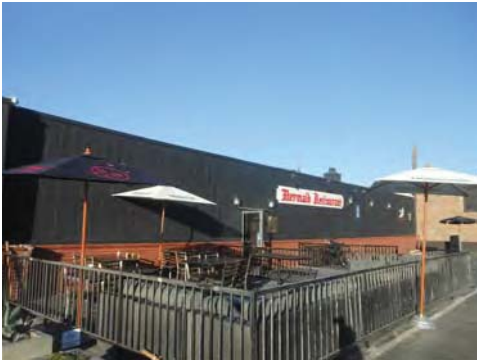
11 Pier Avenue, south elevation
