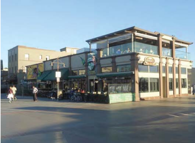
1138 The Strand and 22 Pier Avenue
