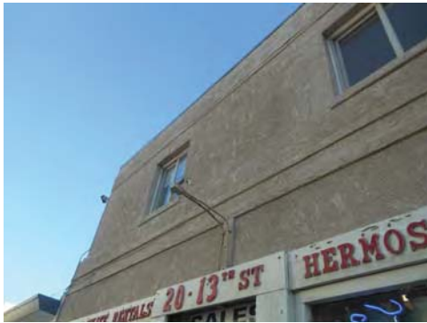
20 13 th Street, exterior finish & window details
