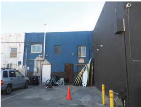
19 Pier Avenue, rear elevation
