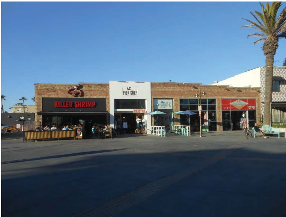
10. 19-31 Pier Avenue, south elevation
