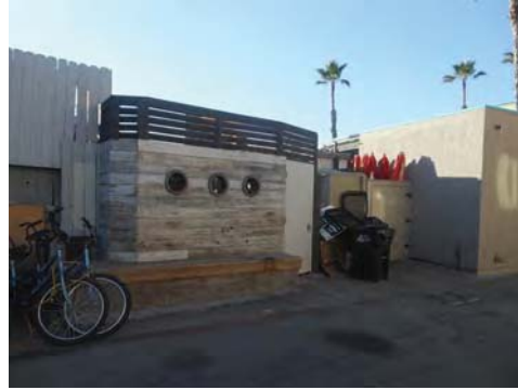
1250 The Strand, rear, east elevation
