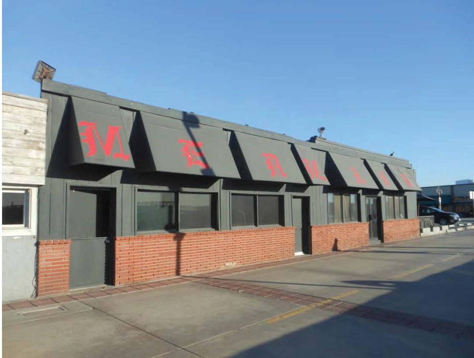
5. 11 Pier Avenue, west elevation
