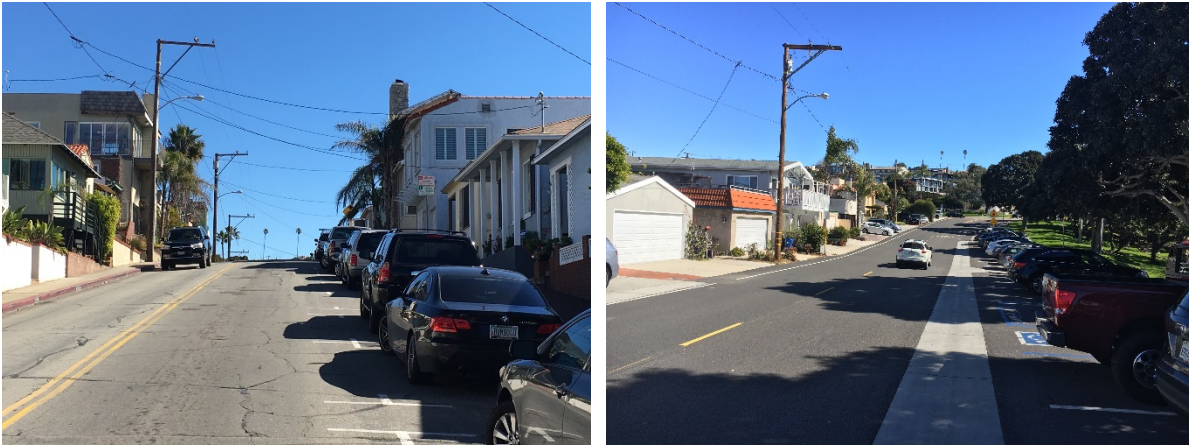
Between Valley Drive and Hermosa Avenue Gould Avenue along the inbound truck route is a narrow 24-foot wide roadway. This segment of Gould Avenue is bordered by residential homes with multiple driveways as well as parallel and head-in parking spaces along the roadway. This segment also passes by Valley Park, which is heavily used by local residents. Crosswalks are provided at Valley Drive and Morningside Drive; however, pedestrians often use the roadway taking a shorter path to the park across the street, or walking on the street to access their vehicles.
