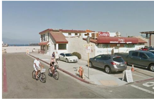
11 th Street adjacent to the south of Scotty's at The Strand provides views of the wide sandy beach and Pacific Ocean.
