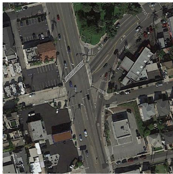
The intersection of Aviation Boulevard & PCH has an adequate turning radius to support haul trucks making left turns onto PCH. However, this intersection currently operates at LOS F, and therefore, the addition of haul trucks could result in substantially increased delays.
