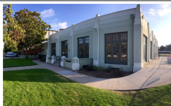
The Clark Building is a historical resource listed on the California Register. The Clark Building is a multi-purpose hall that has a maximum capacity of 240 and is currently used for community classes, meetings, and small gatherings.
