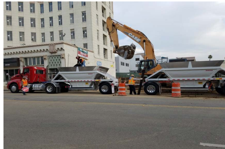
Loading with Excavator
