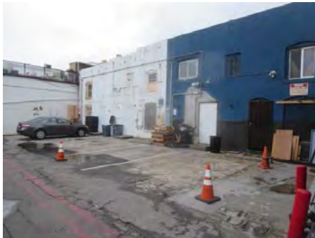
PARKING LOT BEHIND THE SOUTHWEST MULTITENANT SUBJECT PROPERTY BUILDING, LOOKING SOUTHEAST
