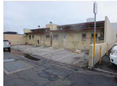
PARKING LOT BEHIND THE NORTH APARTMENT BUILDINGS, LOOKING NORTHWEST
