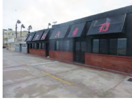
WEST SUBJECT PROPERTY BUILDINGS, THREE RESTAURANTS, LOOKING NORTHEAST
