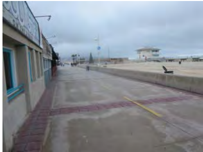
WEST SUBJECT PROPERTY BORDER LOOKING SOUTH FROM THE NORTHWEST CORNER
