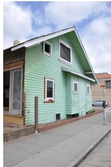
Figure 10: East façade, looking northwest.
