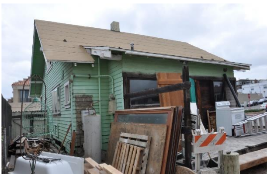
Figure 12: West side of the south (rear) façade, looking northeast.
