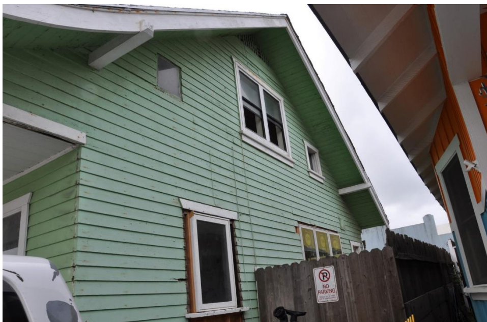
Figure 14: West façade of 70 10 th Street. View facing southeast.
