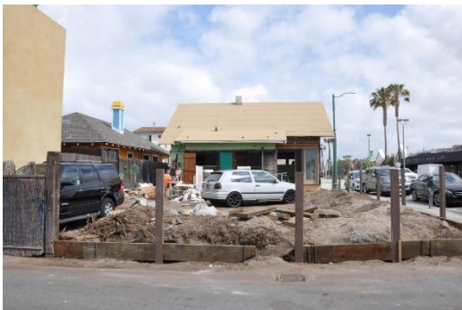
Figure 16: Large rear yard, looking north.
