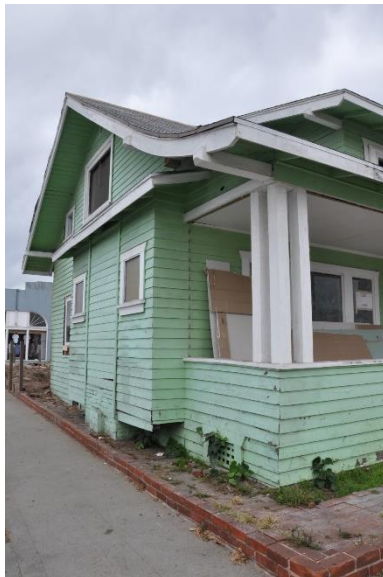
Figure 9: East façade projecting bay with bricks at the ground, looking southwest.
