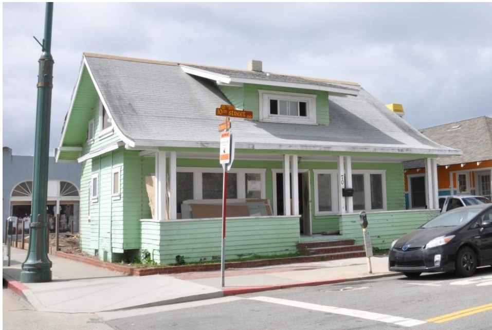
Figure 4. The front (north) façade of 70 10 th Street, looking southeast.
