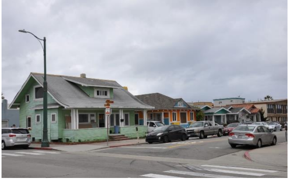
Figure 37: South side of 10 th Street with grouping of five beach bungalow, looking southwest.
