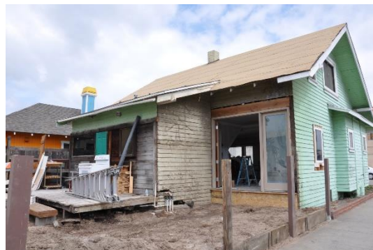
Figure 13: East side of the south (rear) façade, looking northwest.
