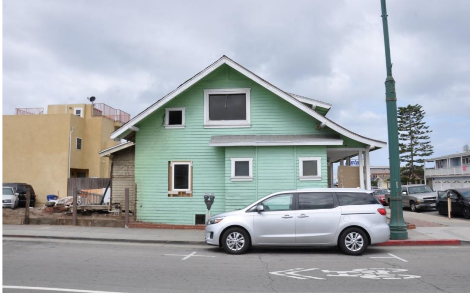
Figure 8: East façade of 70 10 th Street along Hermosa Avenue. View facing west.
