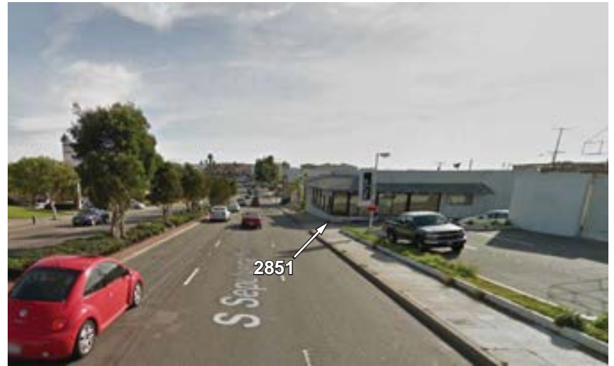
Photo 2: View looking south at 2851 Pacific Coast Highway
