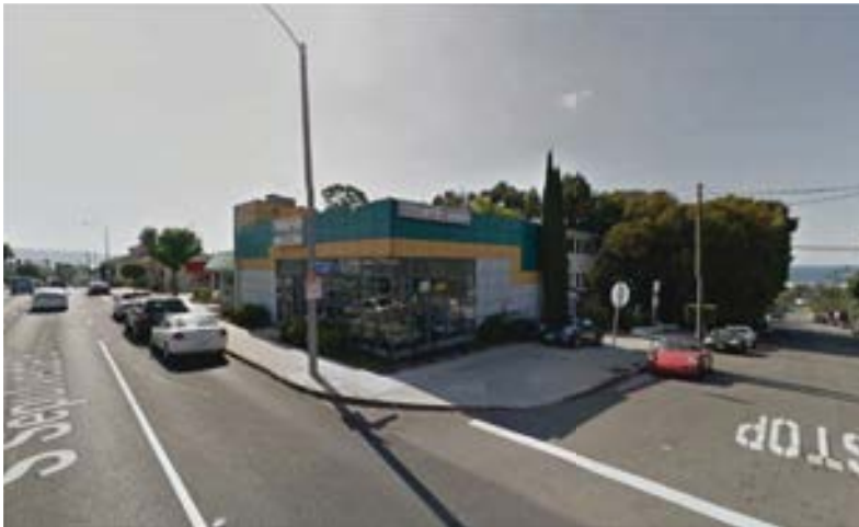
Photo 11: Looking southwest at 317 S. Sepulveda Boulevard
