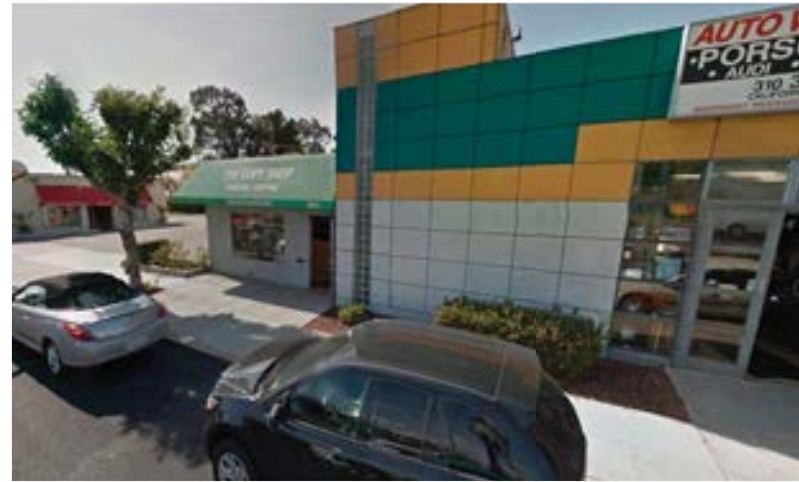
Photo 10: View looking west at 309 S. Sepulveda Boulevard
