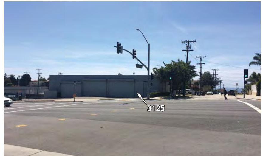
Photo 8: View looking southwest at 3125 Pacific Coast Highway
