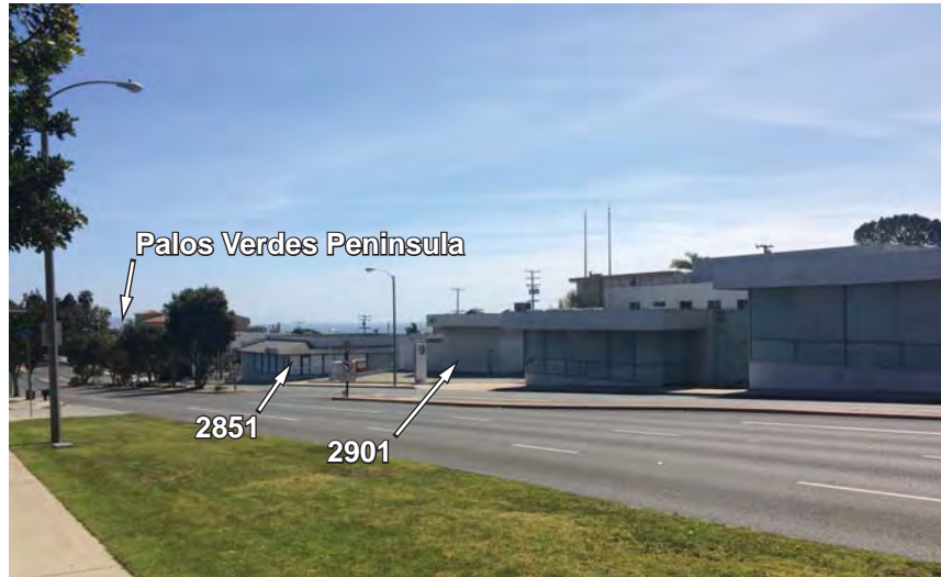
Photo 1: View looking south at 851 & 2901 Pacific Coast Highway
