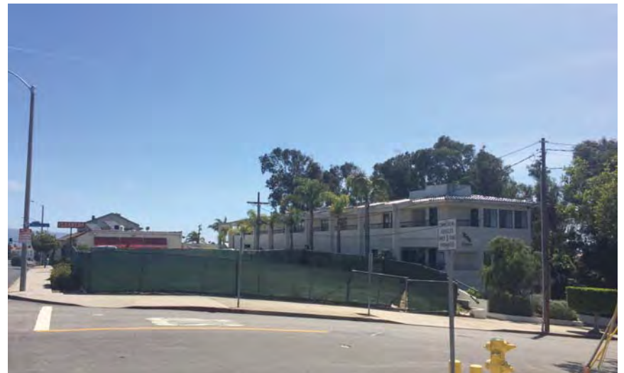
Photo 4: Looking south at 1050 Duncan Avenue
