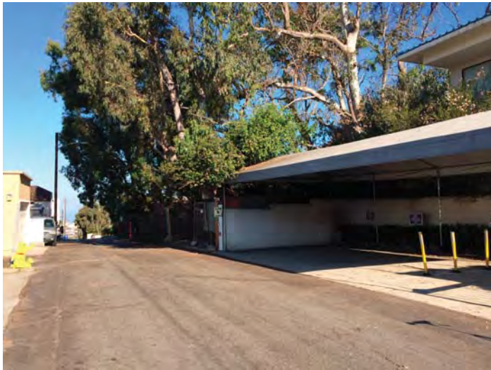
Photo 5: West view of Boundary Place
