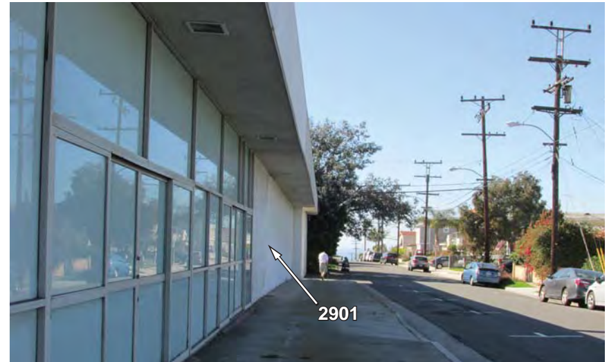
Photo 4: View looking west at 2901 Pacific Coast Highway and down 30th street
