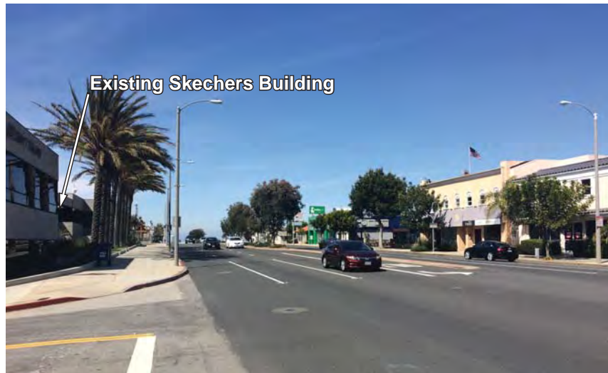
Photo 3: View looking north along S. Sepulveda Boulevard from in between the 305 S. Sepulveda and 330 S. Sepulveda site.
