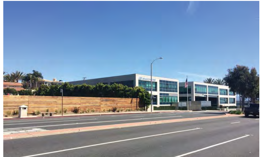
Photo 6: Skechers Buildings south of 330 S. Sepulveda site
