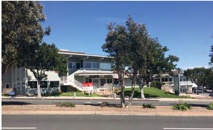
Photo 1: Looking east across SR1 from project site at one- and two-story building on Keats Street and S. Sepulveda Boulevard
