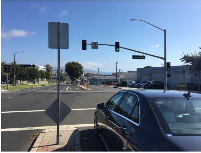
Figure 2. Photographs of views looking south along SR 1
