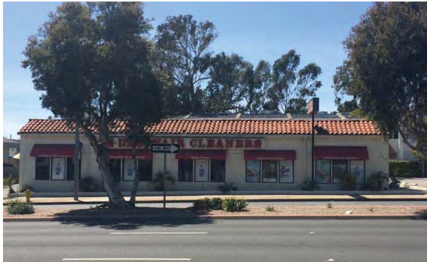
Photo 1: View looking northwest at 305 S. Sepulveda Boulevard
